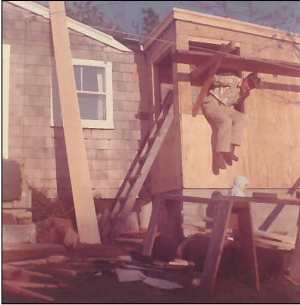
1961 – Work on the cottage addition.
