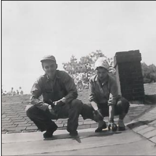
Aleks & Ingrid working on the roof.
