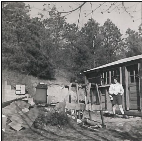
~1959 – Ingrid by the kitchen door. Remodeling has begun.
